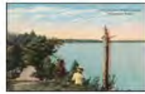
View of East Monposett Lake from White's Island in Halifax
